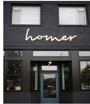
FLAT PANEL BLENDS WITH FACADE
