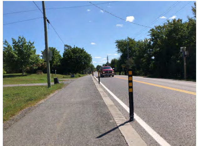
Figure 4-2 | Delineator posts separating multi-use pathway from traffic in the village of Kars in Ottawa
