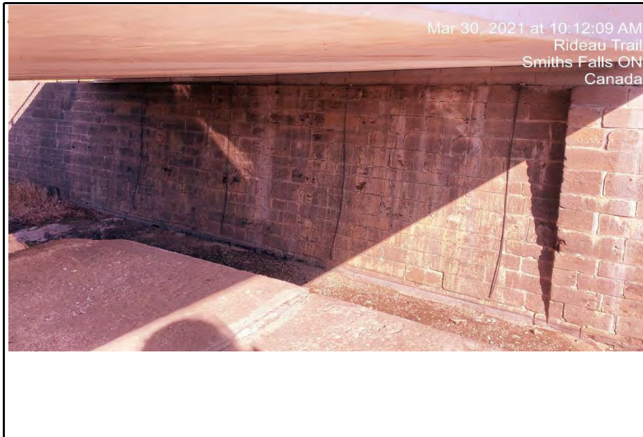
Photo 5: Soffit and Retaining Wall
