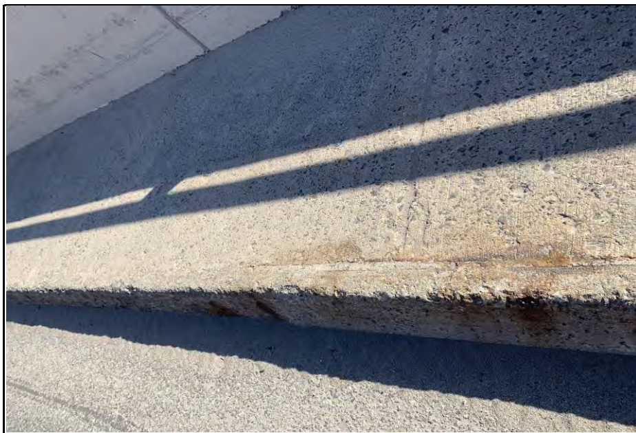
Photo 4: Concrete Curb and Sidewalk
