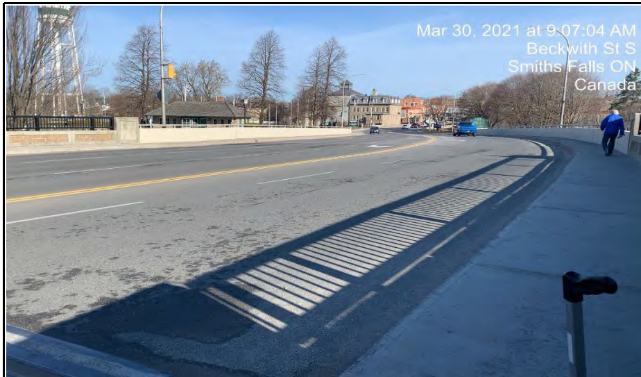
Photo 1: Approach Looking North
