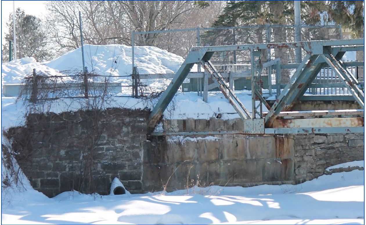
Figure 21: View of the east abutment of the Bridge
