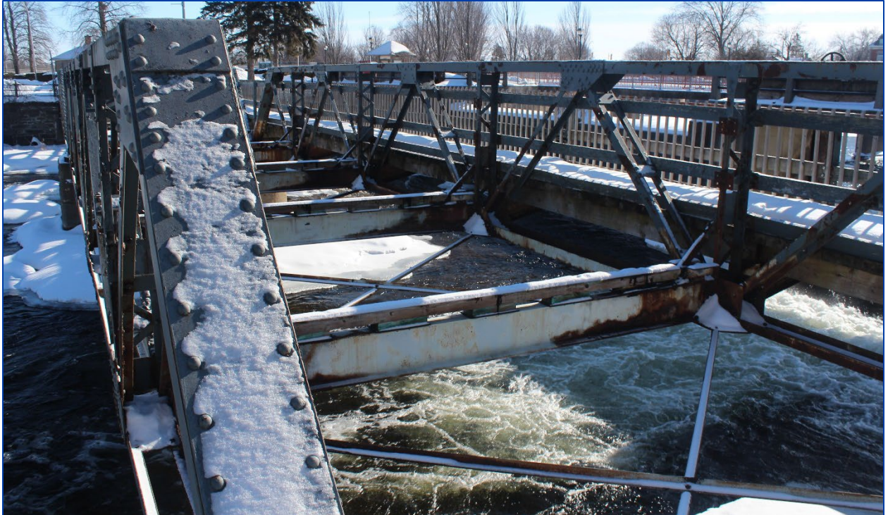
Figure 23: View southeast across the Bridge
