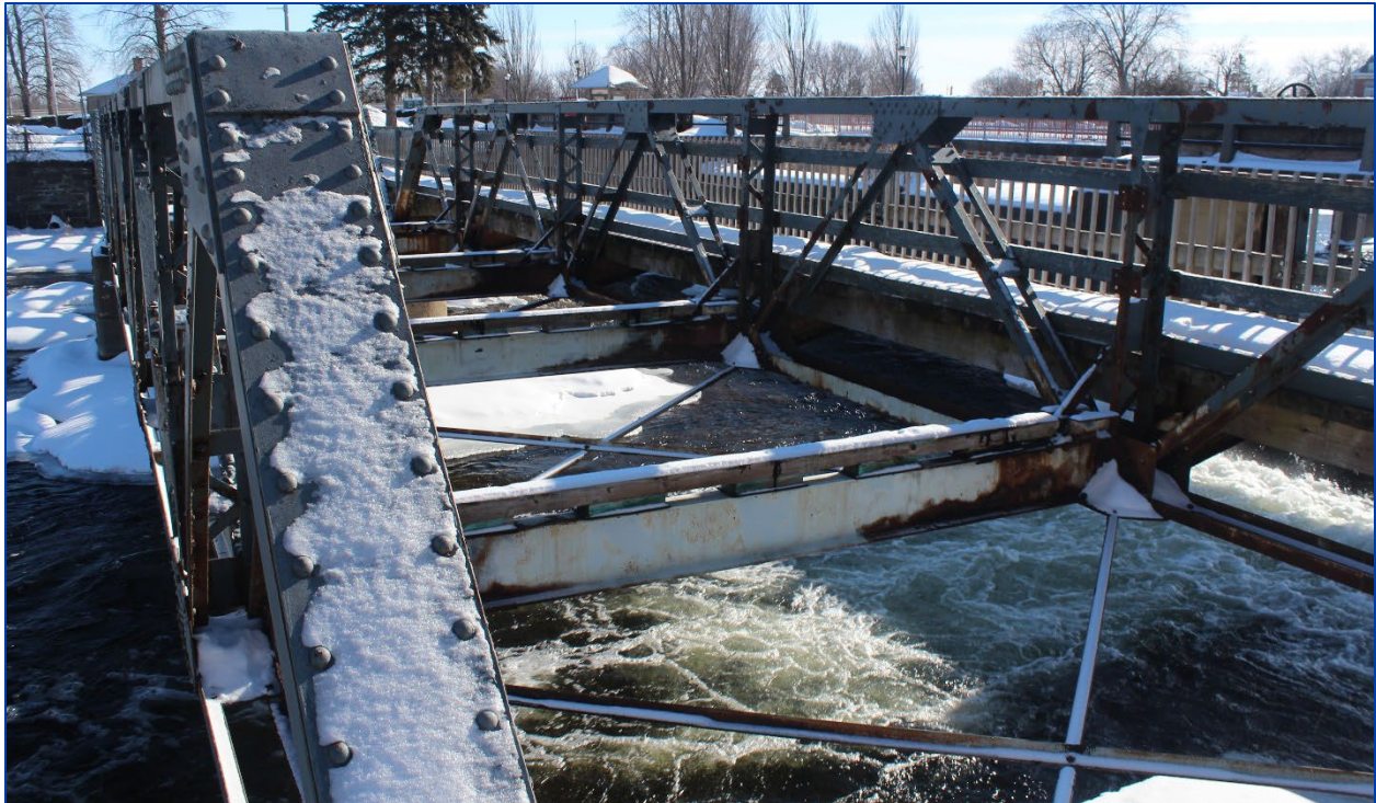
Figure 23: View southeast across the Bridge
