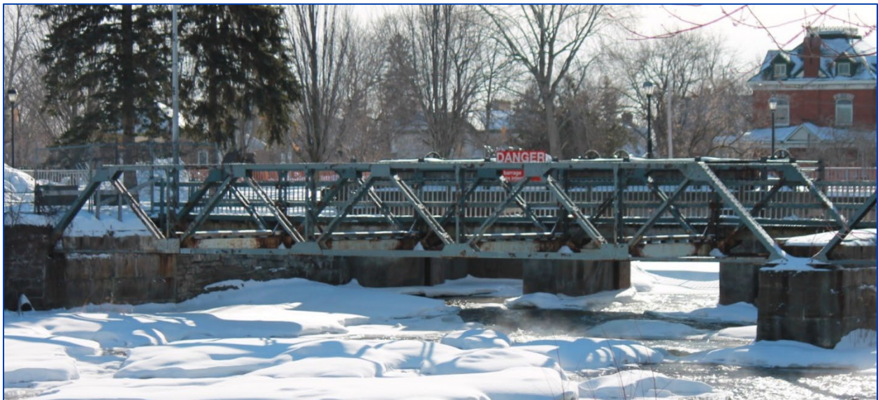
Figure 24: View southeast at the east half of the Bridge
