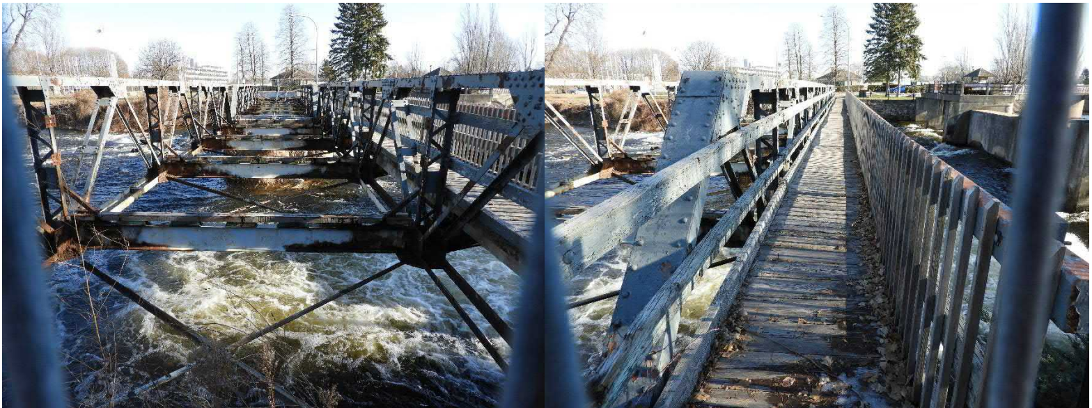
Photo 6: Sections of the Confederation Drive bridge structure where existing timber deck was removed from the bridge (left) and the remnants of the wooden pedestrian pathway (right).
