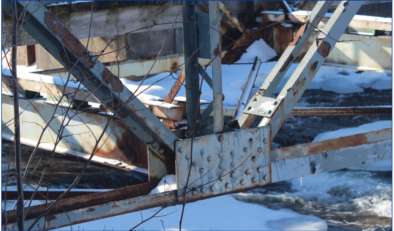
Figure 27: Detail of a gusset plate
