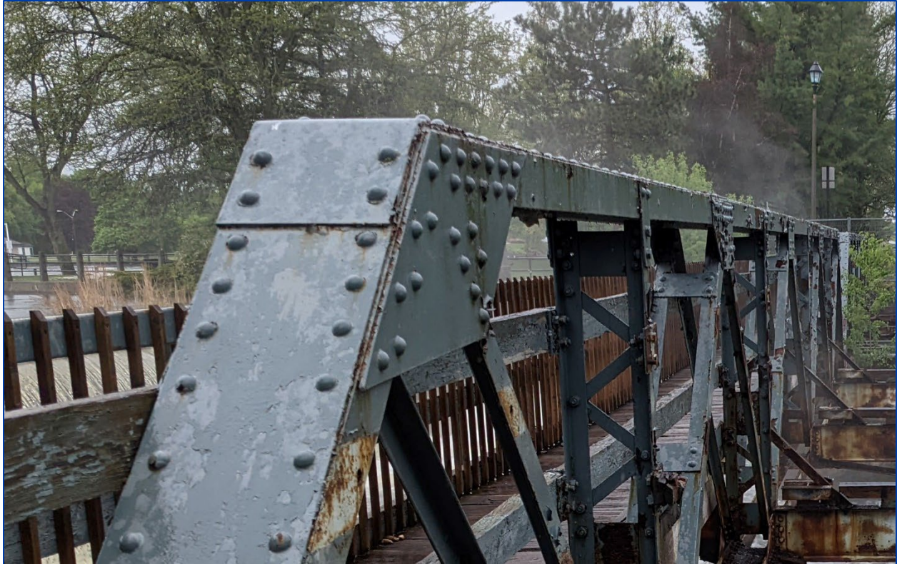
Figure 25: Detail of the top chord construction
