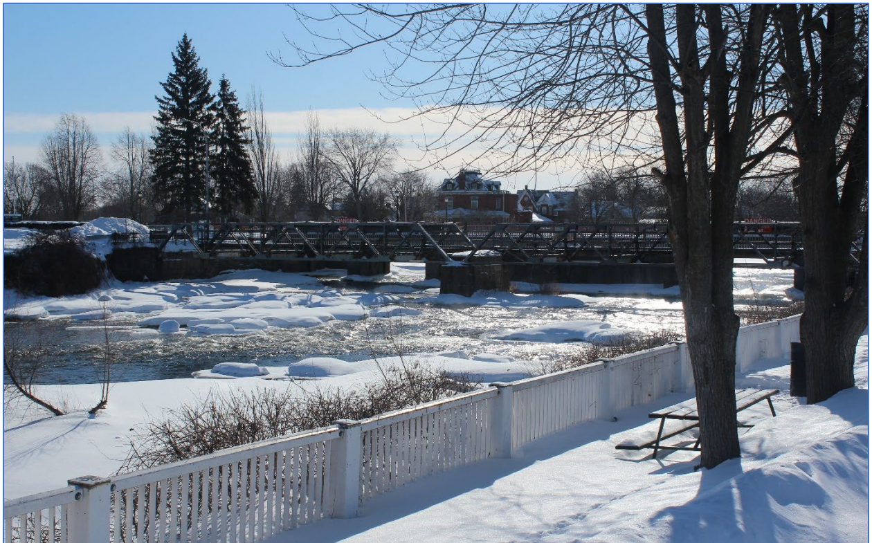
Figure 20: View south of Confederation Bridge
