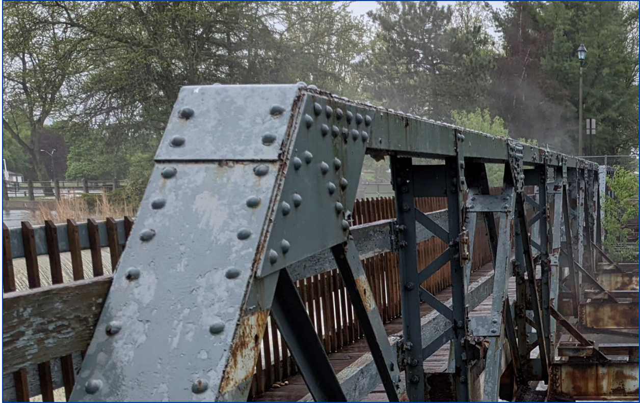
Figure 25: Detail of the top chord construction
