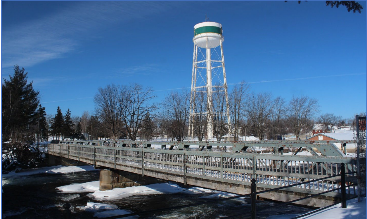
Figure 19: View north of Confederation Bridge
