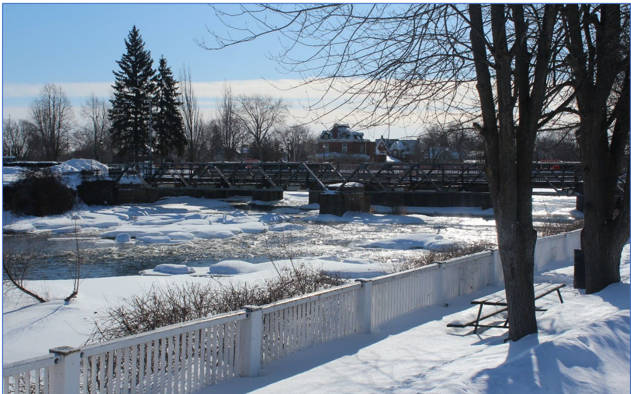
Figure 20: View south of Confederation Bridge
