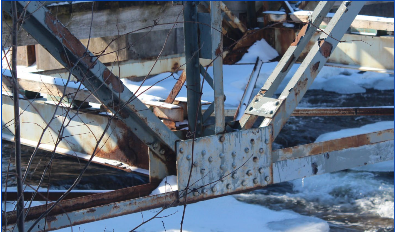
Figure 27: Detail of a gusset plate
