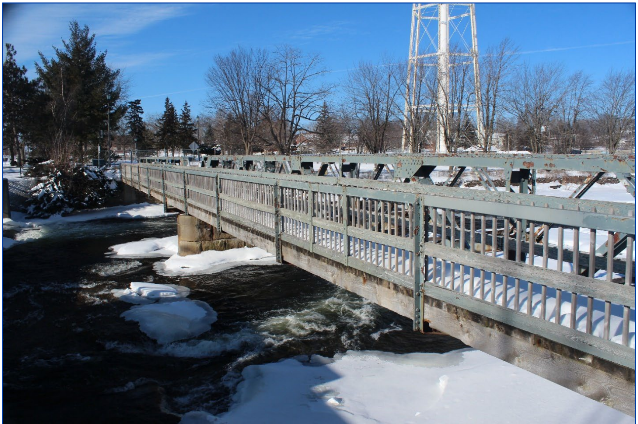
Figure 28: View northwest at the cantilevered pedestrian walkway on the Bridge
