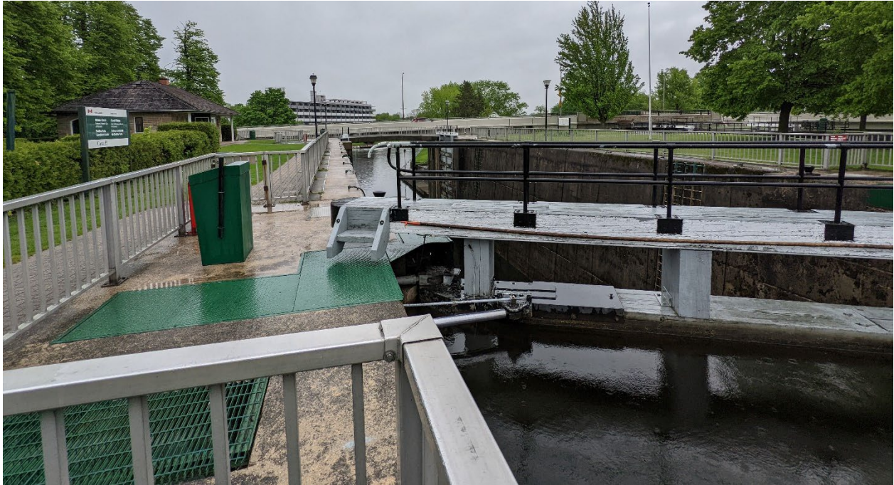
Figure 14: View east at Lock 29a
