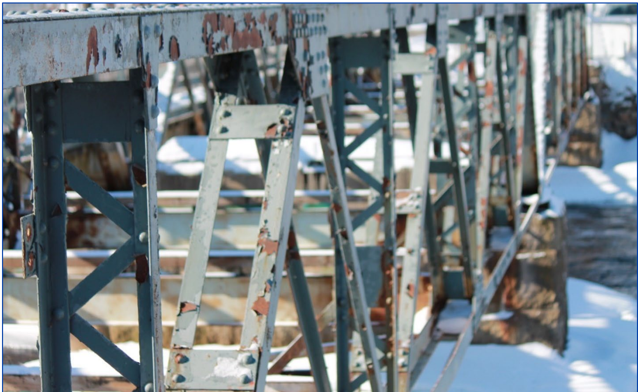
Figure 26: Detail of vertical and diagonal member construction
