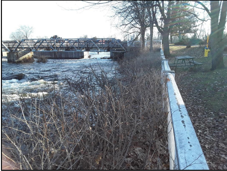
Image 5. View of the Confederation Drive bridge as seen from northwest of the study area, facing south. (PR21-059D002)
