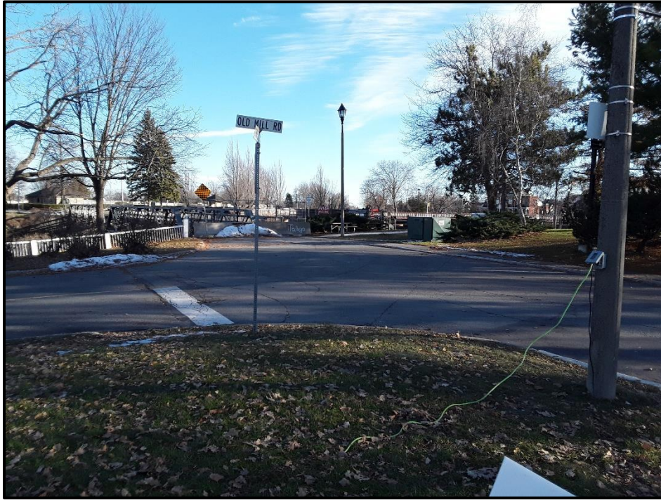
Image 7. View of the Confederation Drive bridge at the intersection of Old Mill Road and Confederation Drive, facing southeast. (PR21-059D005)
