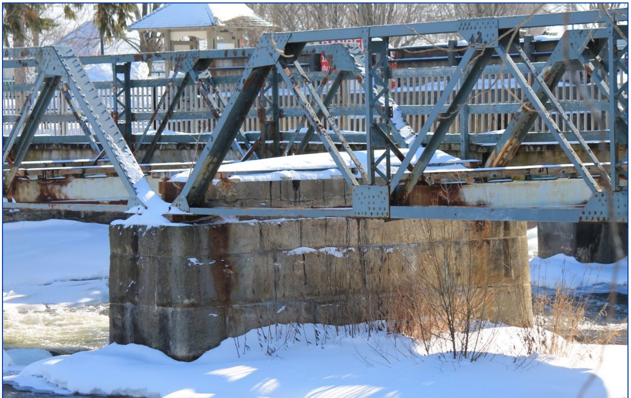
Figure 22: View southeast at the Bridge pier
