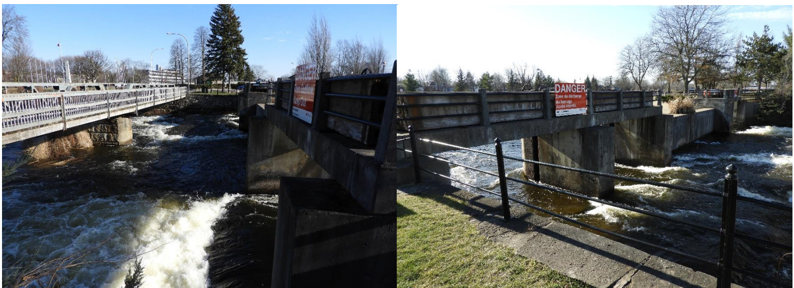
Photo 4: View of the federal dam from the west (left) and east (right) banks adjacent to the Confederation Drive bridge. The presence of this dam creates fast flowing water, which scrubs substrate material and vegetation from the bed of the river and creates large riffles, flats and pools downstream which provides a variety of specialized habitat for several fish species.
