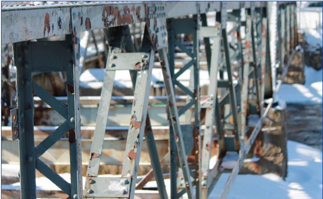
Figure 26: Detail of vertical and diagonal member construction
