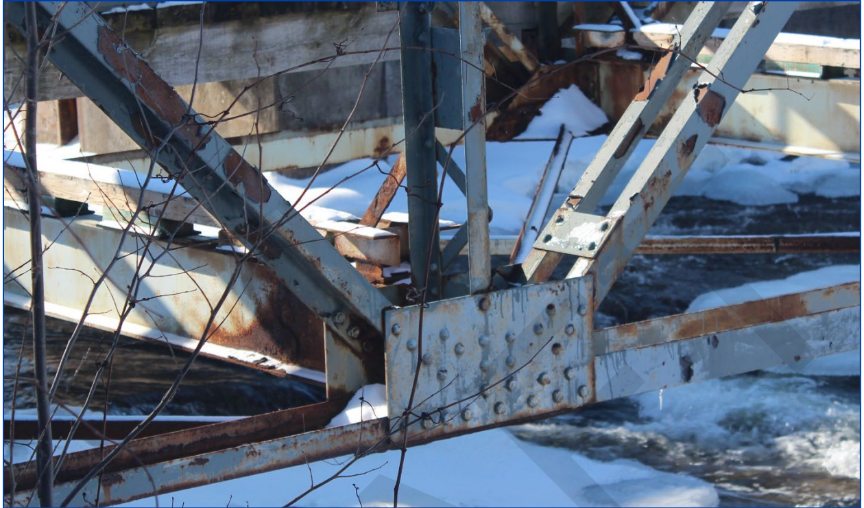
Figure 27: Detail of a gusset plate
