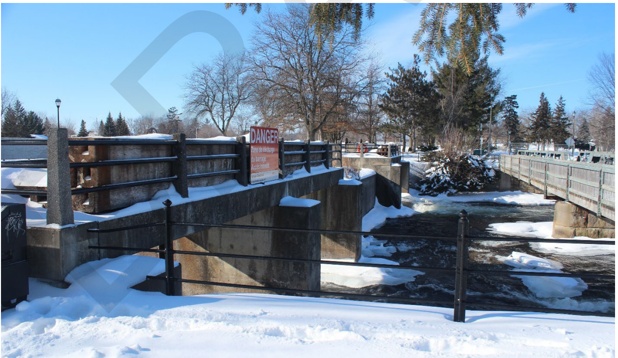
Figure 17: View west at the weir and Bridge
