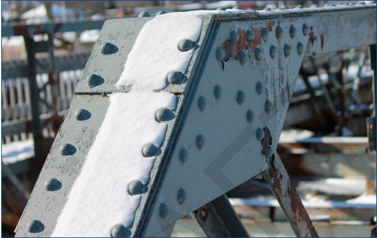
Figure 25: Detail of the top chord construction
