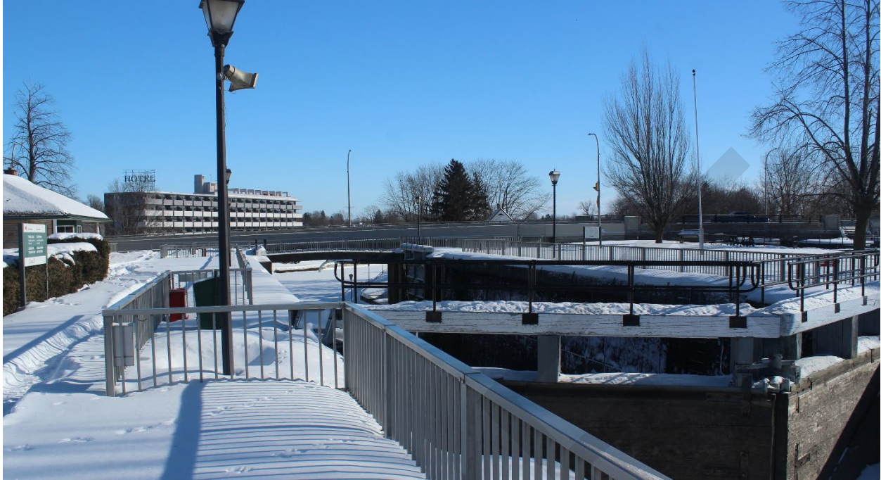
Figure 14: View east at Lock 29a
