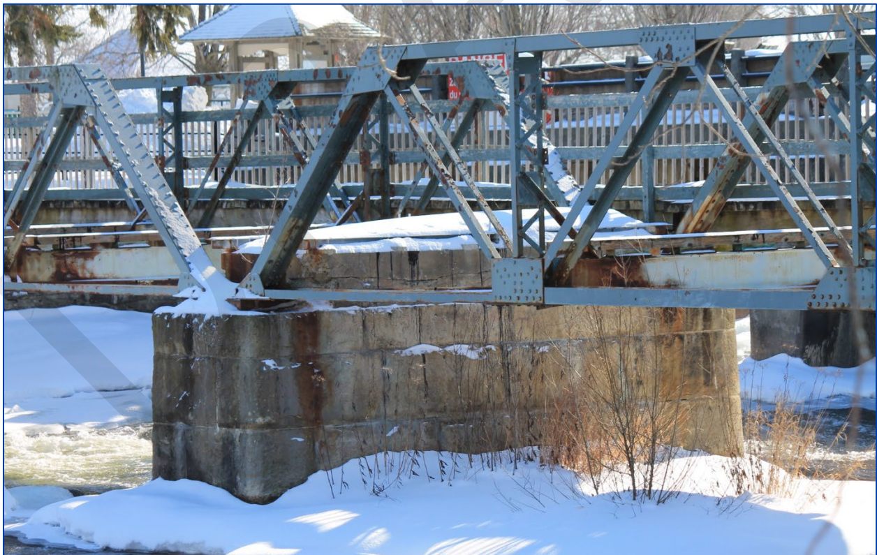
Figure 22: View southeast at the Bridge pier
