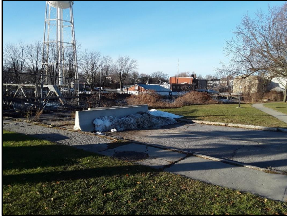
Image 13. View of the Confederation Drive bridge, Canal Street and a manhole cover in the eastern part of the study area, facing northeast. (PR21-059D051)
