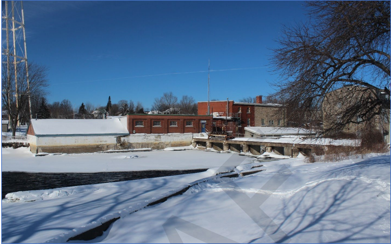
Figure 16: View west of former waterworks buildings on western banks of Rideau River
