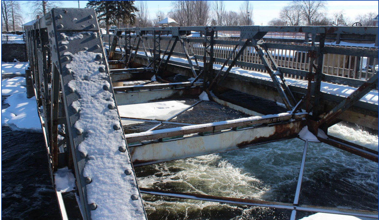
Figure 23: View southeast across the Bridge
