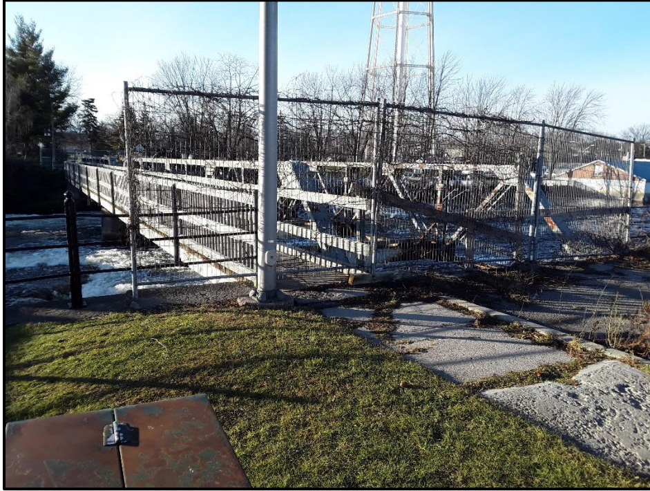
Image 15. View of the Confederation Drive bridge, facing northwest. (PR21-059D074)
