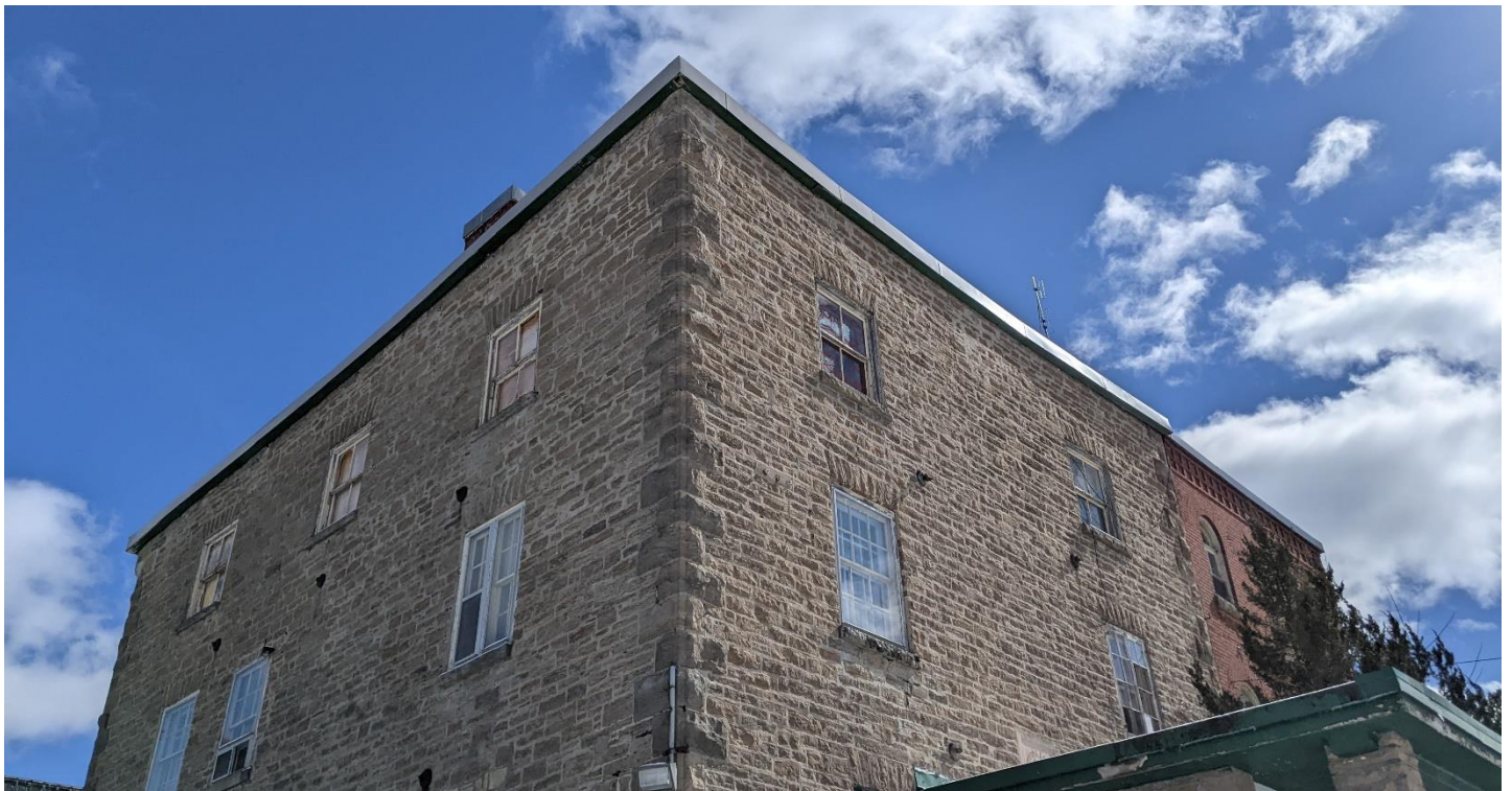
1 Image showing the corner stone quoining on Building 1, and openings, including stone lintels and sills. Image: MTBA.
