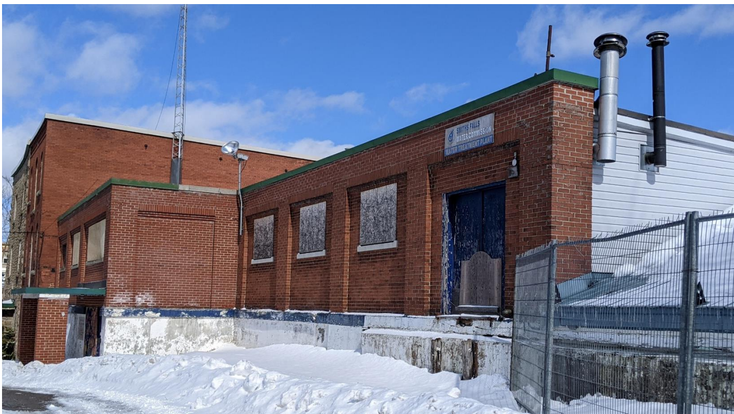
5 Building 3 and its seemingly three distinct rectangular volumes. The first two volumes (left and centre) are two-stories and are constructed of brick. Their geometry and use of brick complements the adjacent Building 2. The openings appear to be recessed within each structural bay, separated by brick pilasters. Each recessed bay has a decorative brick voussoir. The third volume is a basement at the south end of the complex (right), with a metal gable roof. Image: MTBA.
